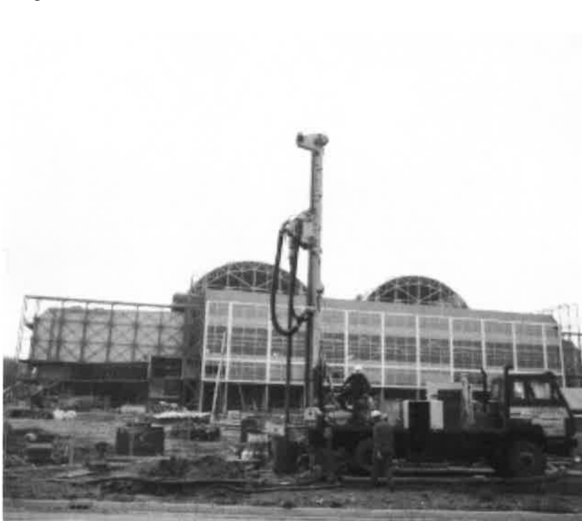
▼ Figure 2: Photo of the Gelredome stadium - installation of ATES.
